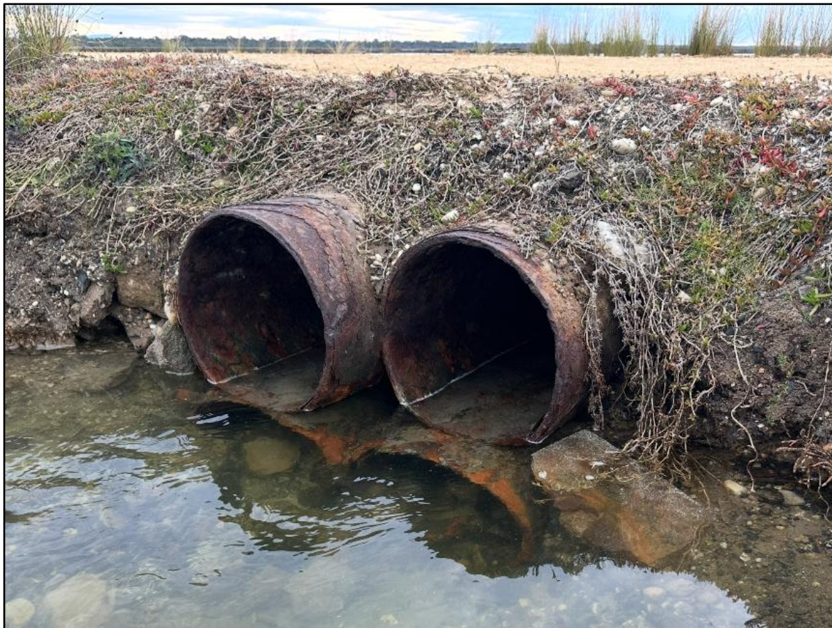
Figure 4: Culverts at the southeastern end of the Track Ten causeway. This is a bank of 4 culverts, 2 upper and 2 lower. Culvert diameter is 430 mm.
