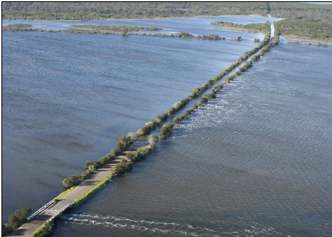
Figure 9: Overtopping of Stockyard Hill causeway 11
