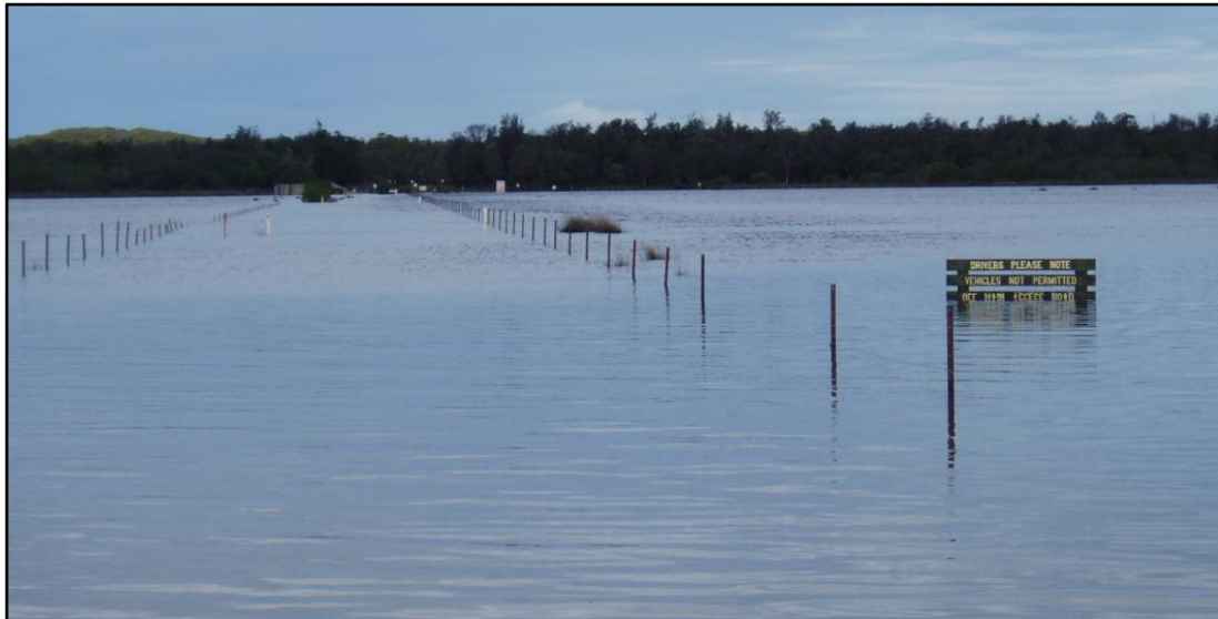
Figure 8: Track Ten causeway 1 July 2007 10 . Water depth is approximately 200 mm deep at the white posts
